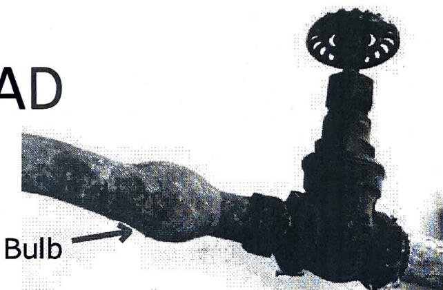
A dull, silver colored pipe that can be easily scratched with a coin or key. Scratching leaves a shiny silver color. Magnets WILL NOT stick to lead pipes. Lead pipes are bendable and commonly have a "bulb".
